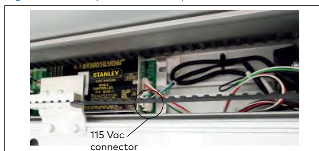
Fig. 3.1.1 Stanley header 115VAC power connection
